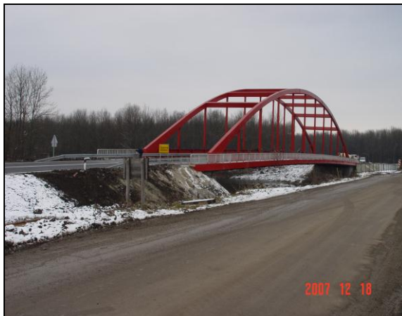
VIEW TO BRIDGE FROM SOUTH - WEST
