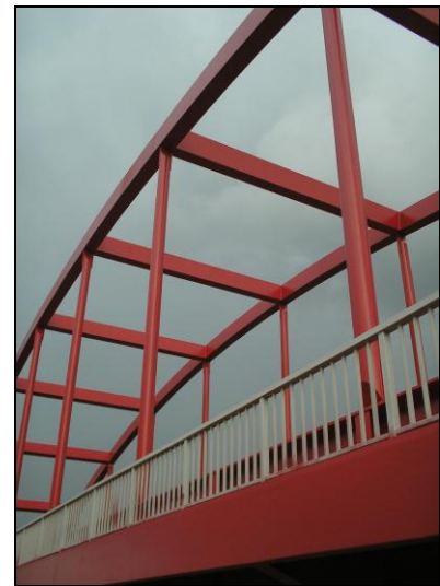
SUPERSTRUCTURE WITH FENCE
