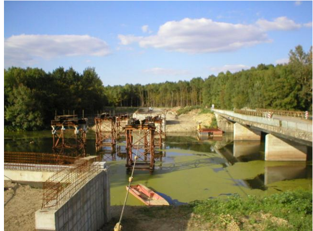
VIEW TO TEMPORARY LAUNCHING PIERS AND OLD BRIDGE
