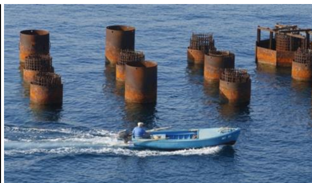
STEEL CASINGS OF PILES DOWN TO 120 M DEPTH
